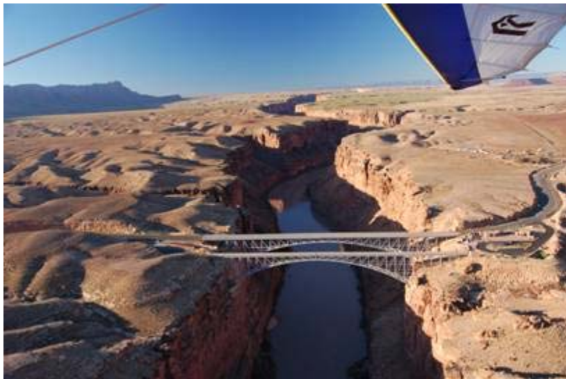
The bridges at Marble Canyon one mile from our camp.
